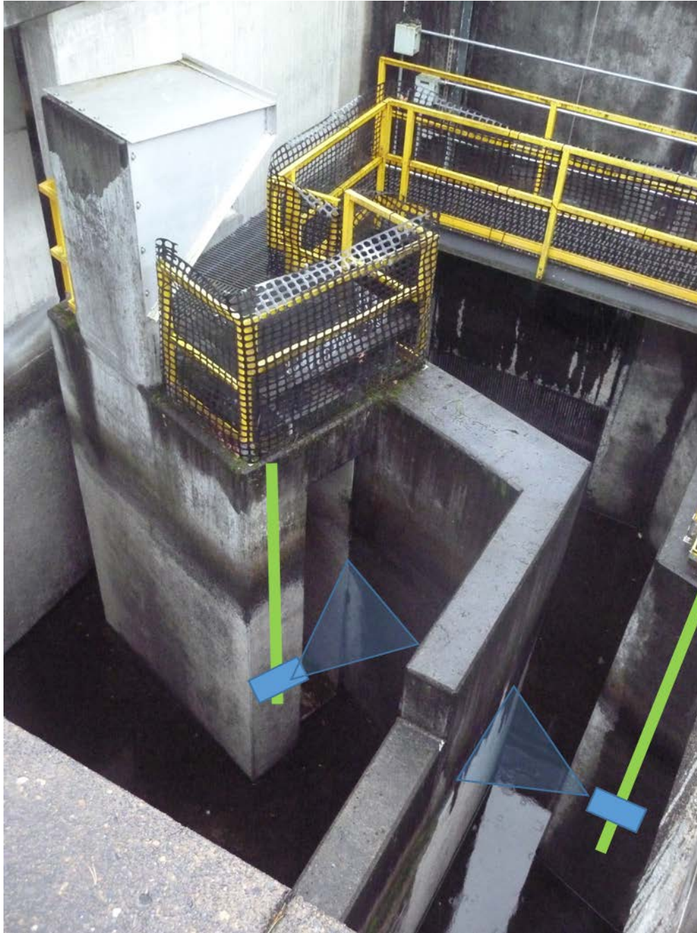
Figure 2: Representative (cartoon) depiction of camera rail and camera deployments in Bradford Island Serpentine Weir section. I-beams sliding in a mounting bracket (green) will support camera and IR light assemblies (blue) during deployment; I-beams and cameras will be removed during non-observational periods.
